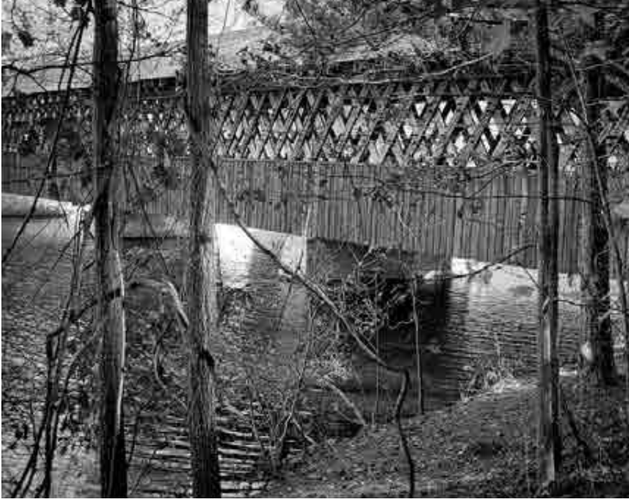
A historic covered bridge crosses to Indian Island.
