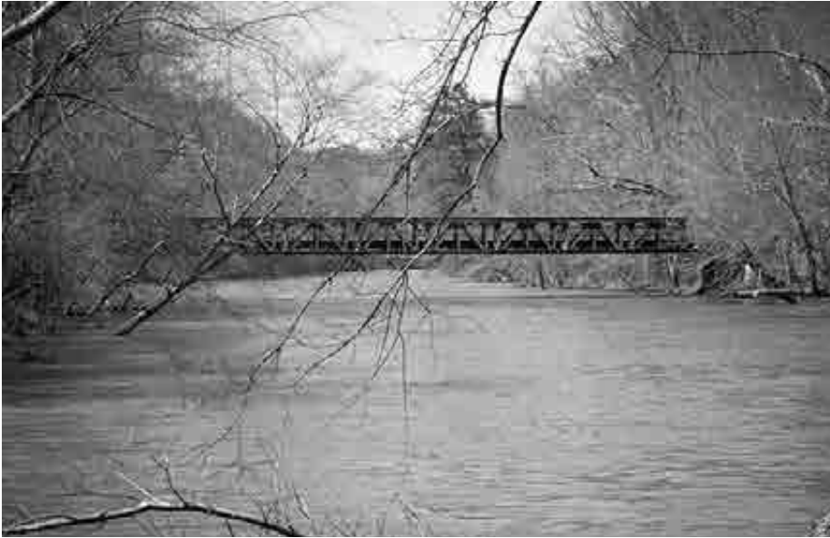
This bridge over Sweetwater Creek was destroyed in the massive floods of 2009. A new bridge, opened in 2012, restored access to most of the Yellow Trail on the east side of the creek.
