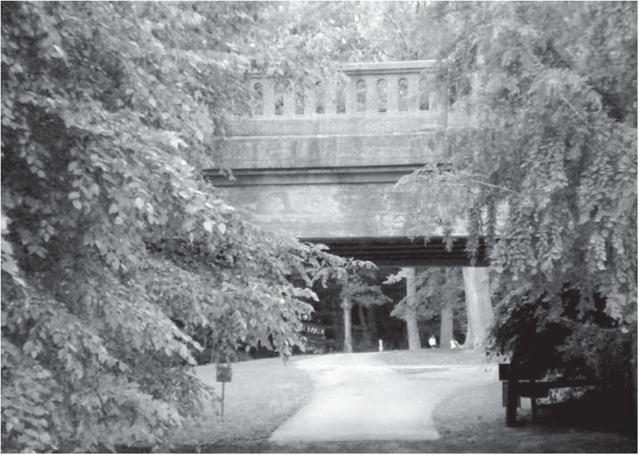
Moredon Road bridge over Lorimer Park trail
